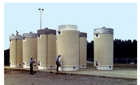
Dry method of storing radioactive waste
